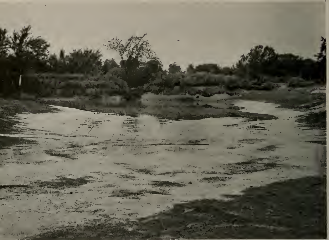
Fig. 4.—The basin of Fork Lake at the time of the dam failure, July 8, 1942. The break in the dam occurred near the center, supposedly as a result of a heavy rain and muskrat tunneling above the normal water line. The bottom of the white exposed portion of the gage board (upper left) marks the former water level.
