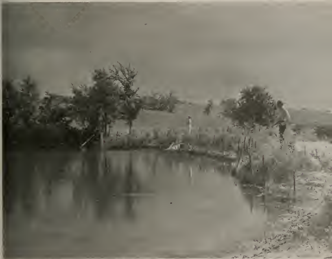
Fig. 3.—Lower end of Fork Lake, showing the dam. Riprapping of broken concrete was held by fencing of wire mesh. This riprapping prevented washing from wave action but was attractive to burrowing muskrats.
