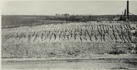
FIG. 2.—Highway cut 7 miles northwest of Kewanee, Illinois. Wp—Peorian loess; Wf—Farmdale loess; It—Illinoian gumbotil and till; Tg—Tertiary gravel; Pc—Pennsylvanian (Canton) shale.
