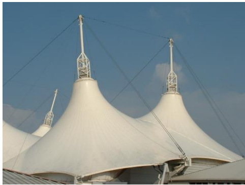
Figure 3: Skyline Pavilion, Butlins, Skegness, UK
