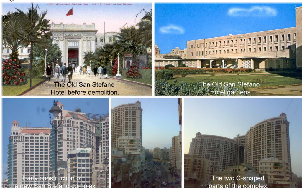
Figure 4: Photos depict the old San Stefano Hotel & Casino and the New San Stefano Towers built on the ruins of the old one
