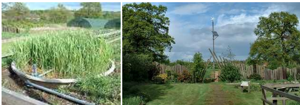
Figure 5 Water Recycling System and Wind Turbine at the Birmingham Park [14]
