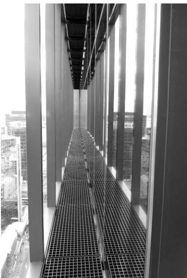
Figure 5: Building B Cavity
