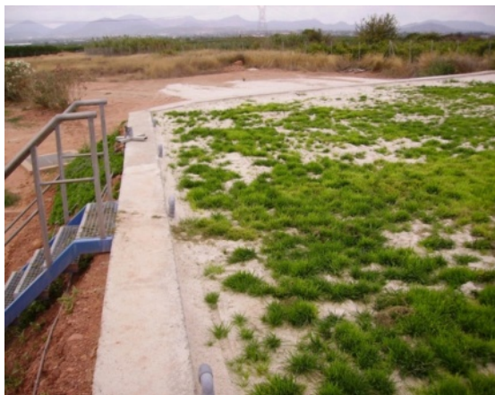
Figure 3. View of the infiltration-percolation system.
