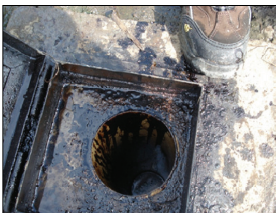
Figure 30. Presence of hydrocarbons into monitoring Well (PM19)
