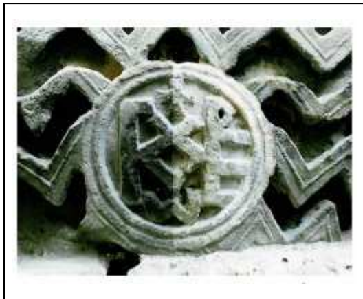
Figure 7. A laser cleaned section from the outdoor decoration of the 12 th century church of Panaghia Kapnikarea in the historical centre of Athens (Marakis, 2000) [62]. The application was carried out with the 3rd harmonic of the Nd:YAG laser (355 nm) using consecutive pulses at 0.4 and 0.5 J/cm 2 .
