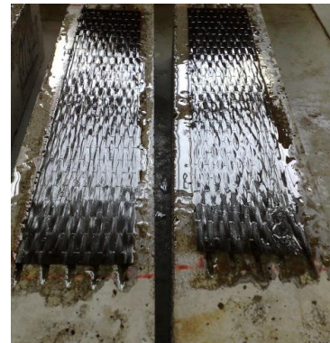
Figure 8 – Wet lay up CFRP application
