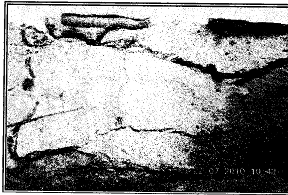
Fig. 9. Crushing of concrete (top-side view) of Beam 2-2
