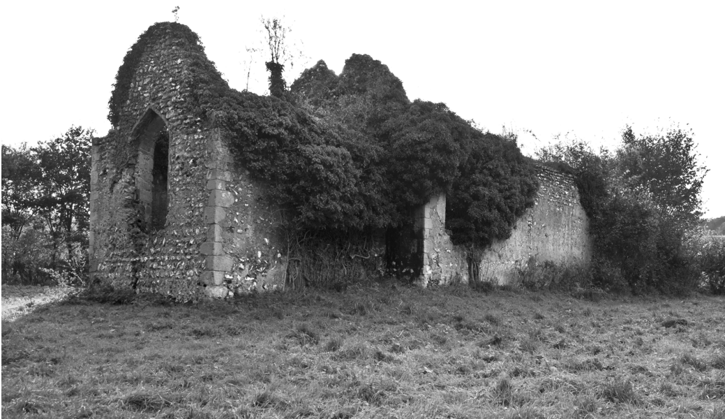
Fig. 2. The ruins of Bix Brand church, looking south-west, 2009. This is a two-cell Romanesque structure with late-medieval and subsequent alterations. The nave may have been extended. Photograph by Derek Kendal. © English Heritage. NMR, DP074742.
