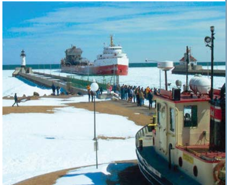
Duluth jetties, Minnesota: Transfer of the Duluth harbor from St. Paul District to Detroit District took place in 1979. (Photo by Casandra Brewster, courtesy of Detroit District, Corps of Engineers)
