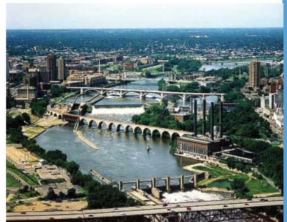
Upper and Lower Locks at St. Anthony Falls, Minneapolis: The falls were the highest point of navigation on the Mississippi River when the Corps of Engineers opened an office in St. Paul in 1866. (Photo courtesy of St. Paul District, Corps of Engineers)
