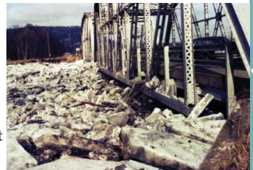
Ice Jam on the Root River, 1982: Ice jams are one cause of frequent floods in the shallow river valleys of northwest Minnesota and northeast North Dakota. (Photo by Lyle Nicklay, courtesy of St. Paul District, Corps of Engineers)
