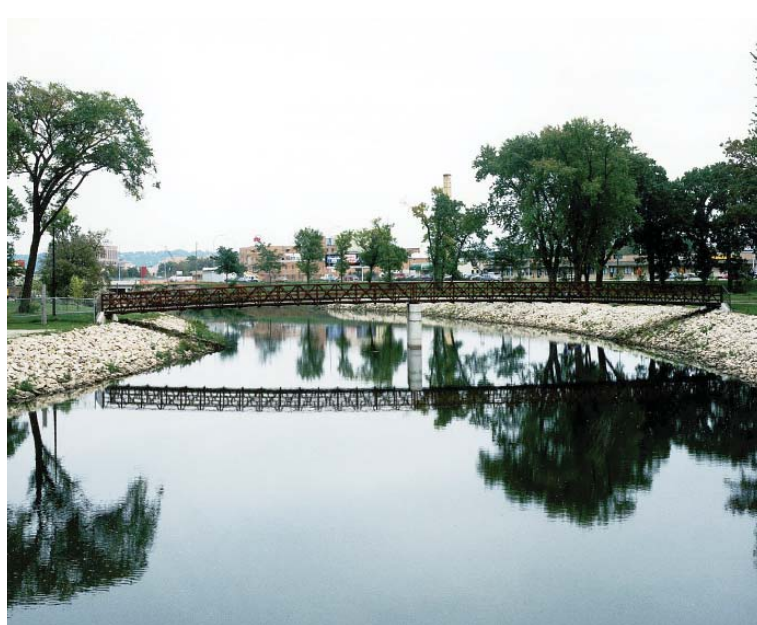
Zumbro River: Channel modifications on the South Fork Zumbro River in Rochester, Minnesota, showing the pedestrian bridge and riprap implemented by the St. Paul District, 1995. (Photo courtesy of St. Paul District, Corps of Engineers)
