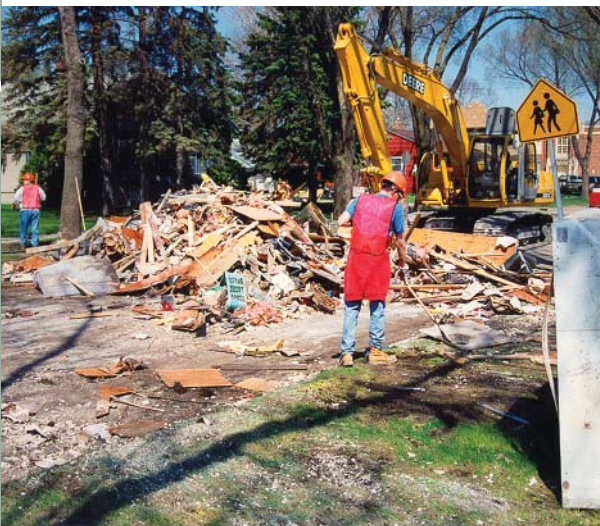
Cleanup: Corps' contractors cleanup the aftermath left in Grand Forks, North Dakota, by the devastating Red River of the North flooding in 1997. (Photo courtesy of St. Paul District, Corps of Engineers)
