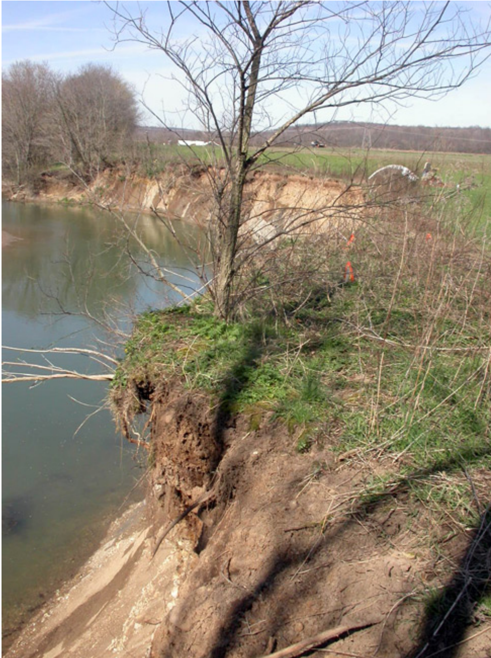
Figure 3 Erosion along the southern edge of site 33RO1059.
