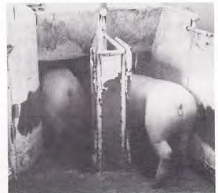
Figure 4. A wedge-shaped partition installed between the two single-file chute entrances prevents jamming. The wedge enables one hog to pass another.
