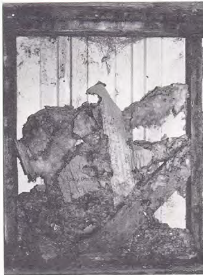
Figure 1. Fiberglass batt insulation within walls of a hog finishing house was destroyed by house mice in less than three years.
