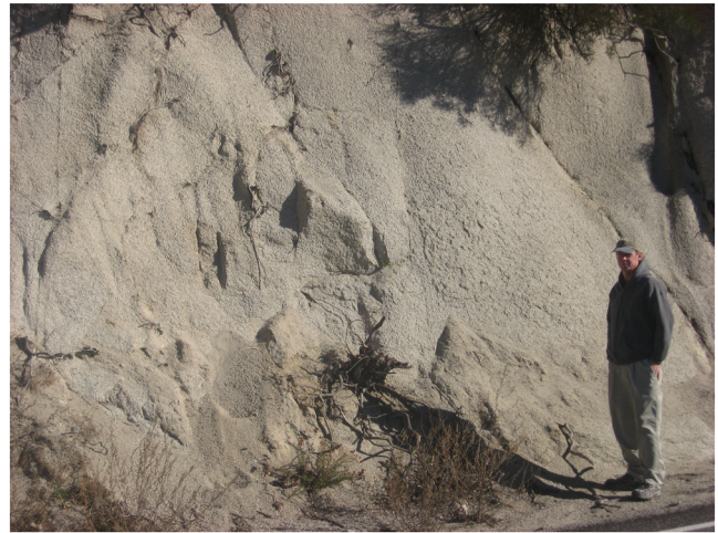
Figure 3. Granitic saprock in the San Jacinto Mountains in southern California. Note roots protruding from joint fractures. Rock matrix can be easily excavated with hand pick, knife, or spade, but individual minerals show little sign of chemical alteration. Exposed section is about 5 m thick; man in photograph is 1.85 m tall.
