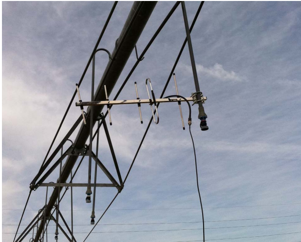
Fig. 4: An aboveground mote attached to the center-pivot.
