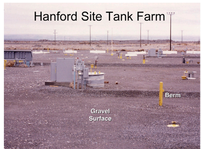
FIG. 4. Bare surfaces at a Hanford tank farm.
