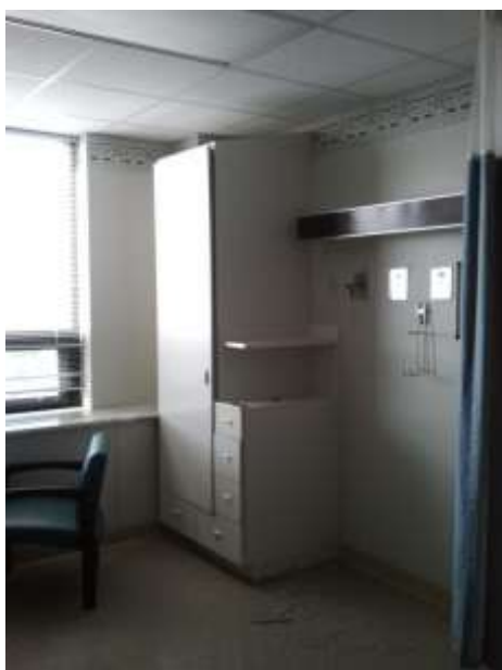
Figure 7-Shared patient room prior to remodeling.
