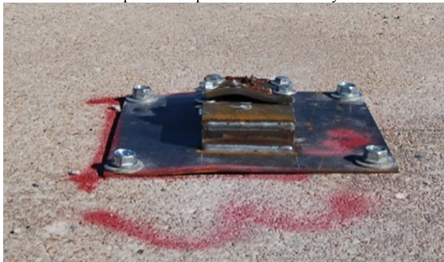
Upstream Slip Base Post Assembly
