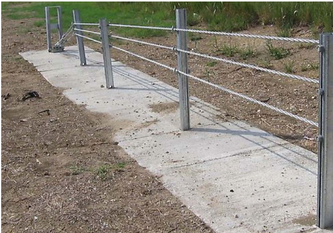
Figure 5. Gibraltar End Terminal
