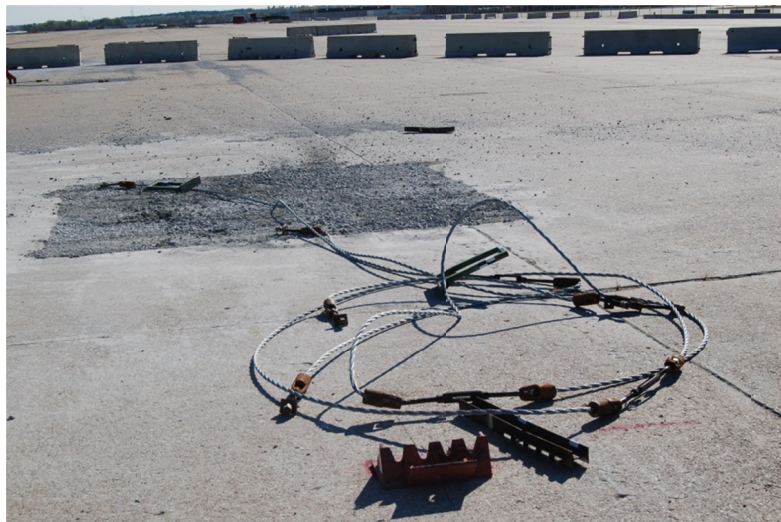
Figure 52. System Damage, Test No. HTCT-1
