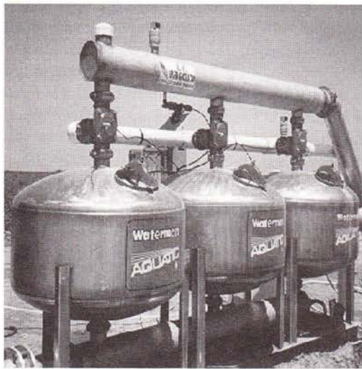
Figure 5. Photo and schematic sand media filter (photo courtesy of Waterman Industries, Inc.)
