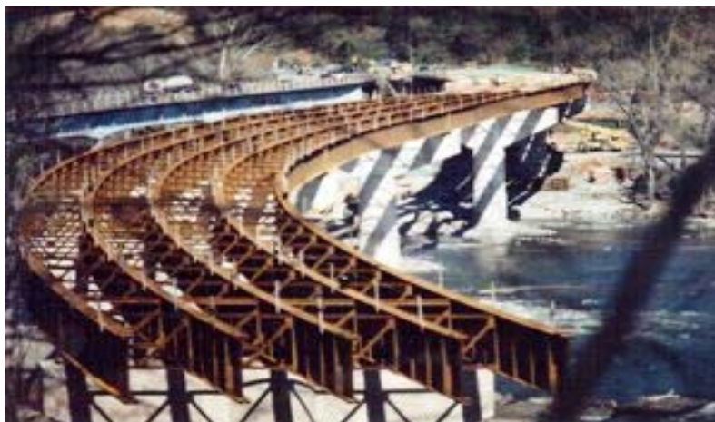
Figure 4.1-1. A Curved Steel I-girder Bridge Similar to the Studied Bridges
