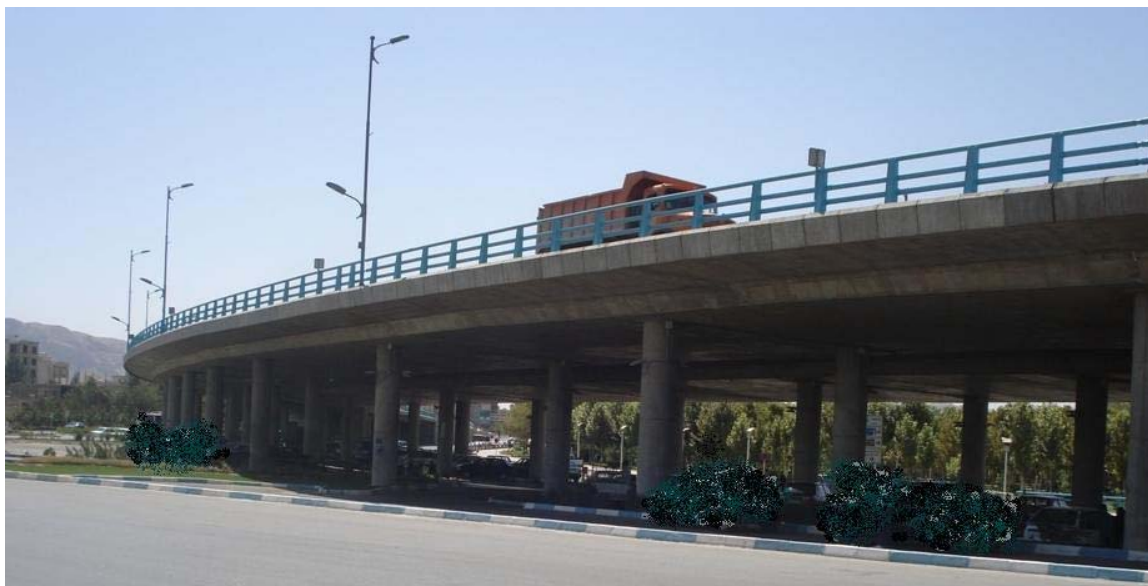
Figure 5.1-1. A Concrete Curved Integral Bridge Similar to the Studied Bridges
