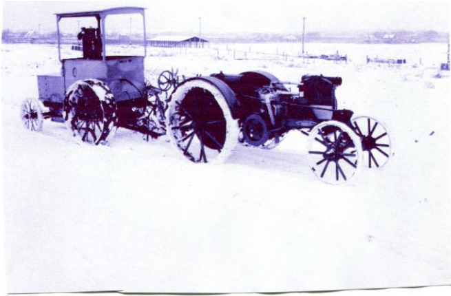
Figure 43. First tractor test car consisting of an Illinois tractor being pulled in reverse driving the engine in reverse to load the tractor. A Gulley Tractor Dynamometer with a mechanical integrator was used to read and record instant horsepower. This is the first trial, testing a Minneapolis 12-25 tractor. The tractor was withdrawn and re-tested as Test # 12. Testing in snow proved impractical.
