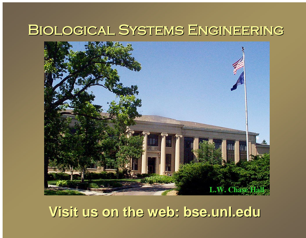
Figure 38. L. W. Chase Hall today. It still fills its designed role as the anchor for East Campus.
