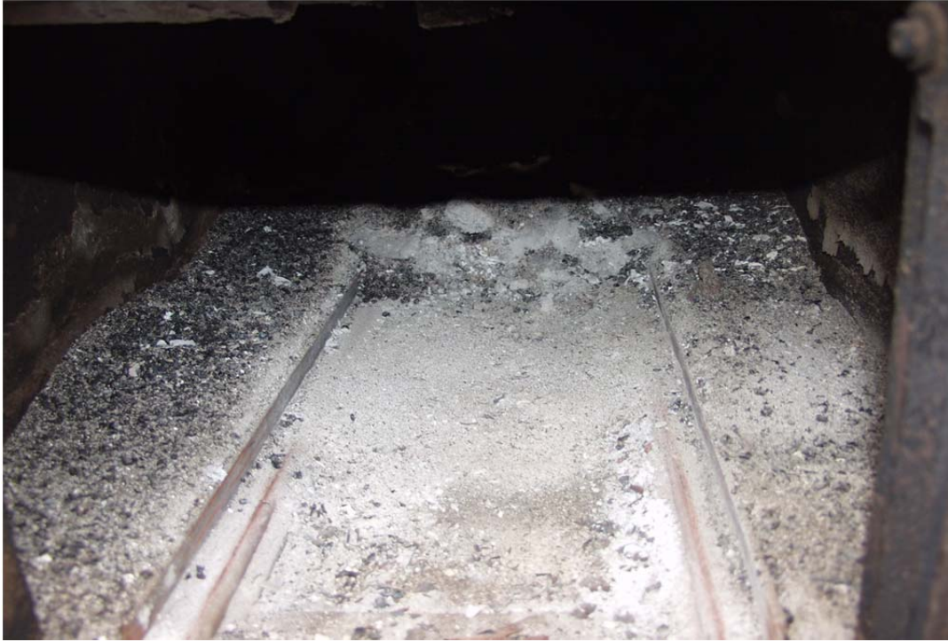
Figure 3.6. Firebox Ash Buildup.
