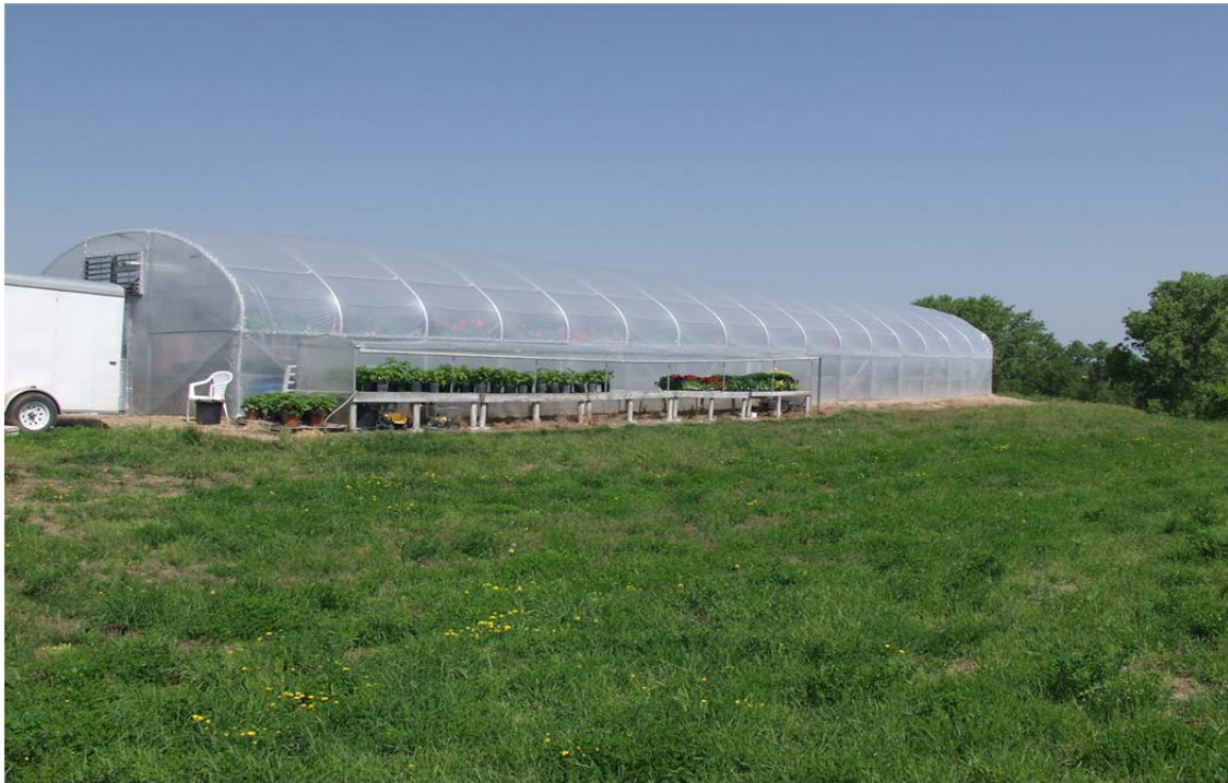
Figure 2.1. Firth Nebraska Cooperator Greenhouse (East side)
