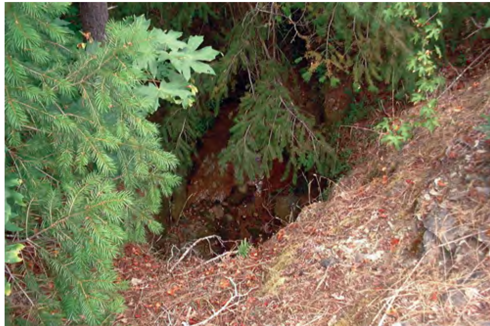
Figure A22. Hunts Hill drainage tunnel outlet, near Buckeye Ford in Greenhorn Creek, Nevada County, California.
