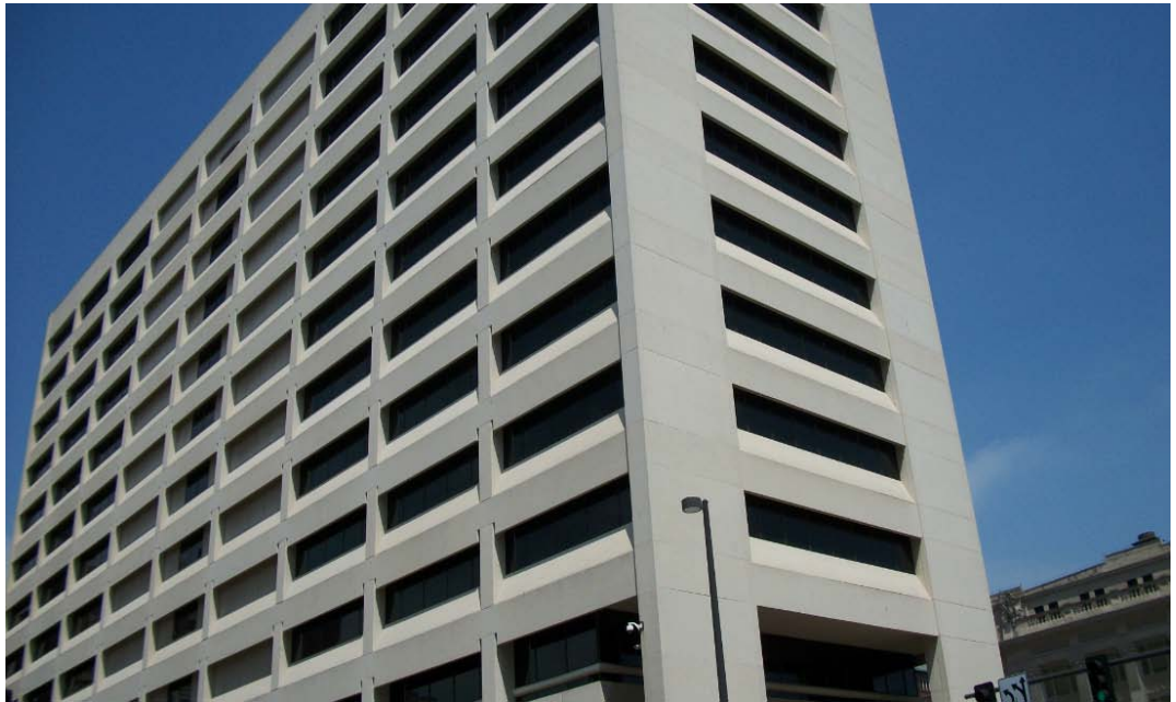
Figure B-0-6: Case building side view
