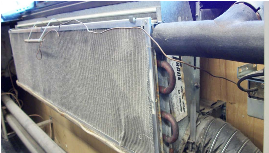
Figure B-0-10: An induction unit
