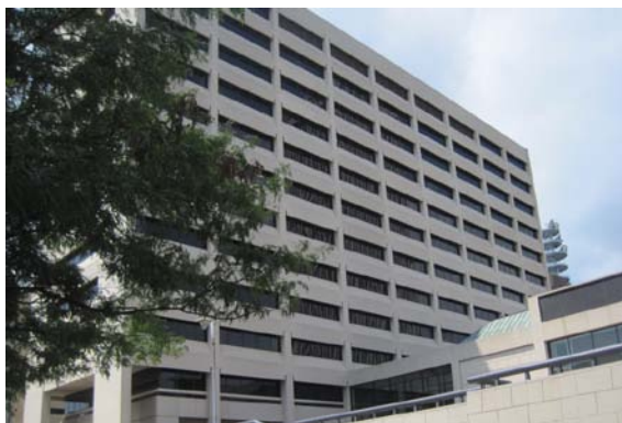
Outside view from south east
