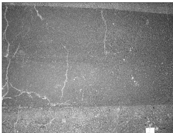
Figure 2.13 - Strong asphalt section built with limestone (White et al., 2006)
