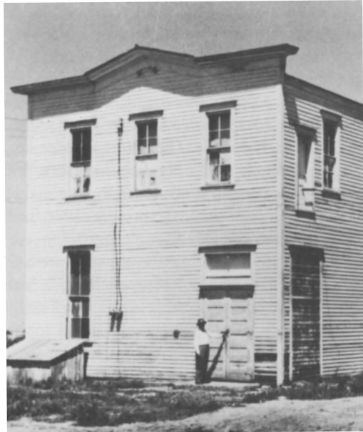
FIG. 10. The opera house in Iroquois, Dakota Territory (South Dakota), was built in 1882. At the time this picture was taken in 1955, the lower floor was a church with the stage hidden behind the pulpit by a wallboard partition. Photo courtesy of South Dakota State Historical Society.
