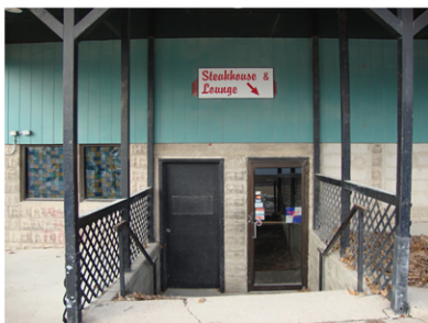
sub-level entrance on south side
