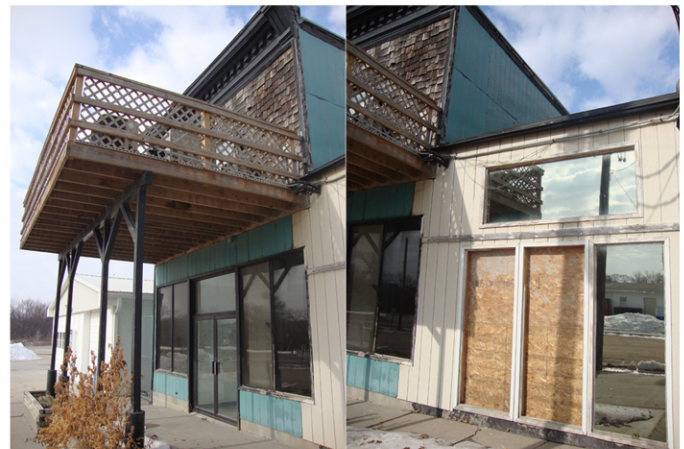
western side of structure
