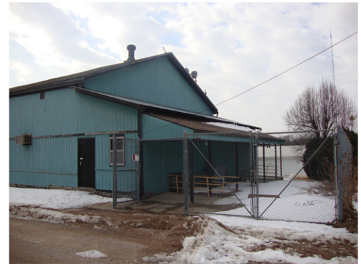
patio facing north: rear facade
