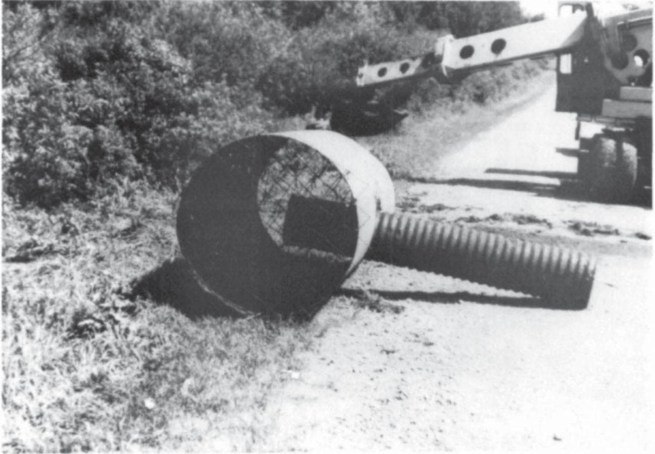
Figure 2. Large culvert showing placement of hole cut for smaller diameter connecting culvert. Wire mesh is in place on culvert ends.
