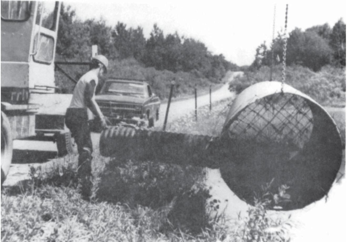
Figure 4. Lowering assembled T-culvert in place in front of road culvert.
