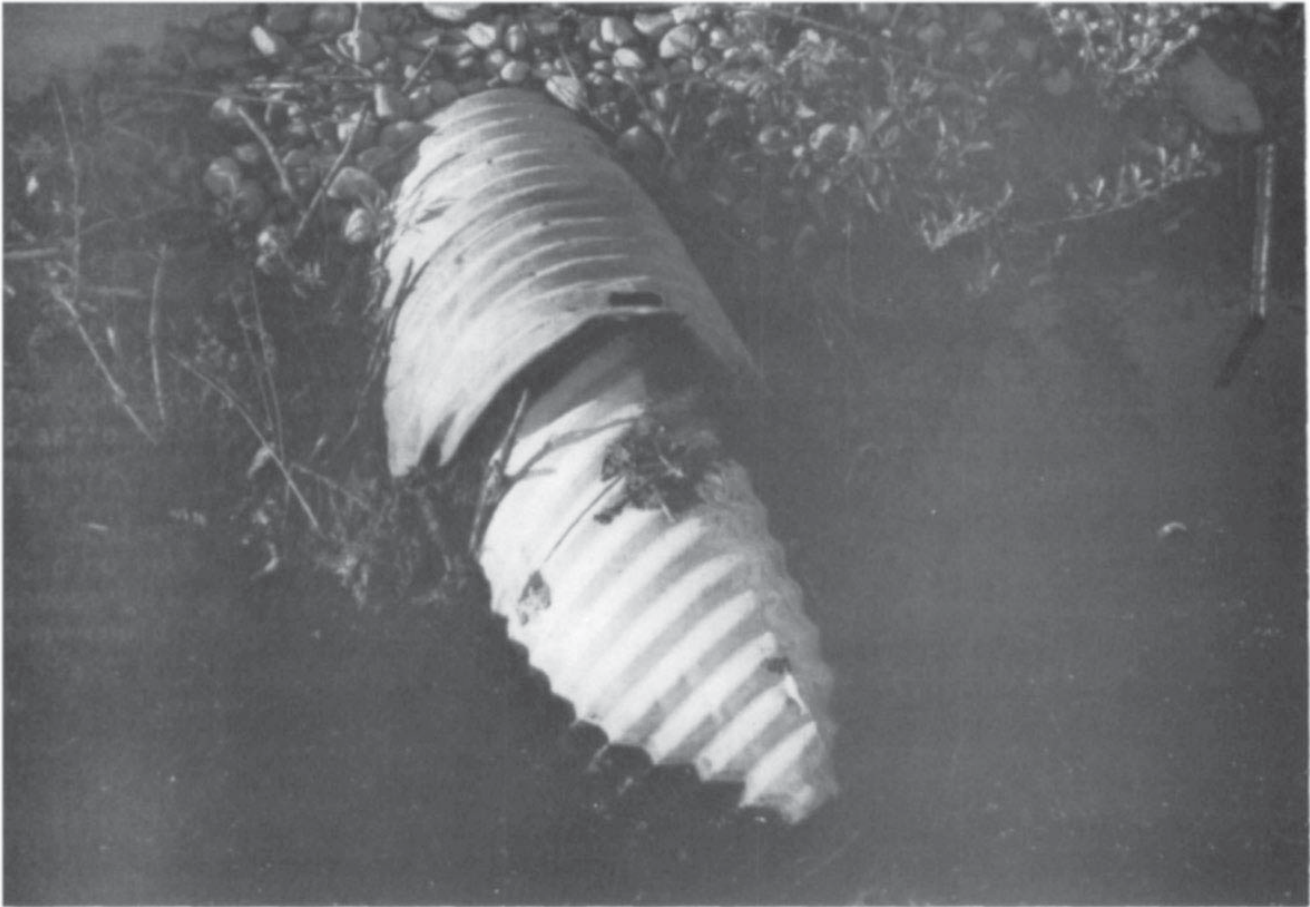
Figure 5. Smaller diameter connecting culvert in place in road culvert.
