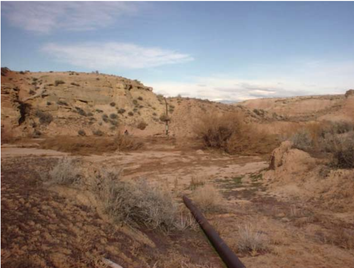
Figure 6. Channel degradation or scour during flash-flood events may expose buried pipelines, resulting in costly breaks.
