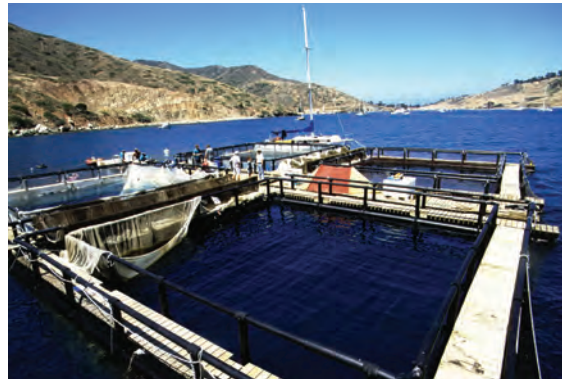
Figure 2.9 An aquaculture net pen offshore of Catalina Island, California, 2000. The walkways provide access for commercial fish feeding and pen maintenance.
