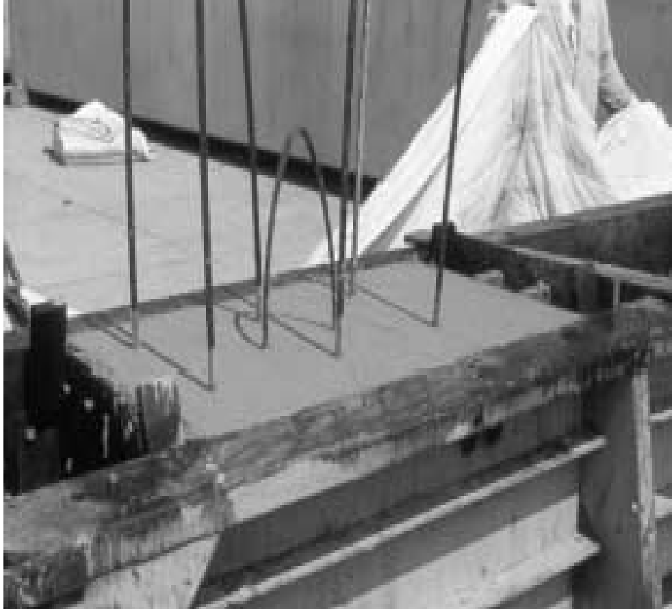
Figure 2.11: Finished pullout test block (Barnes et al. 1999)
