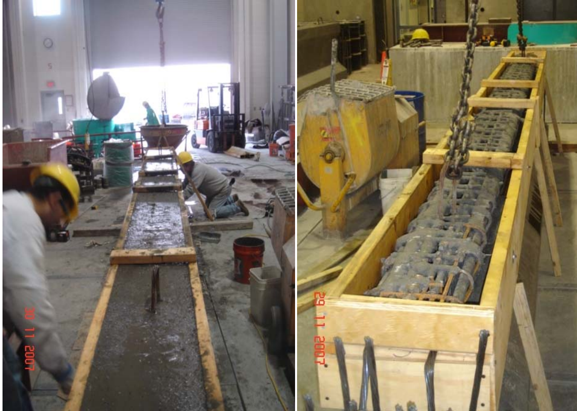
Figure 5.7: Pouring girder B top flange – University of Nebraska Lab
