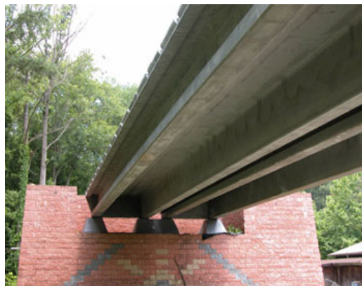
Figure 4.3: Pi-girder bridge at TFHRC
