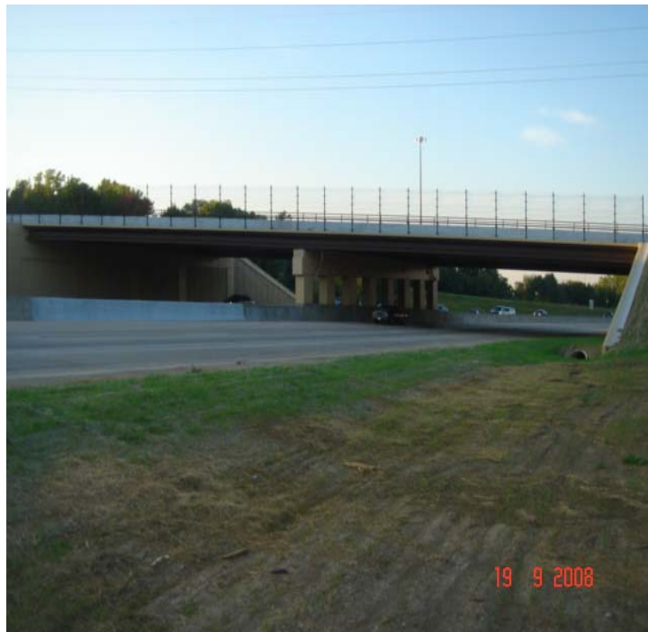
Figure 1.1: Pacific Street and I-680 Bridge, Omaha, Nebraska
