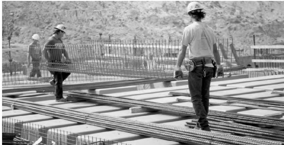
Figure 5.1: Placing a WWR shear cage in a girder (WRI Manual of Standard Practice, 2006)
