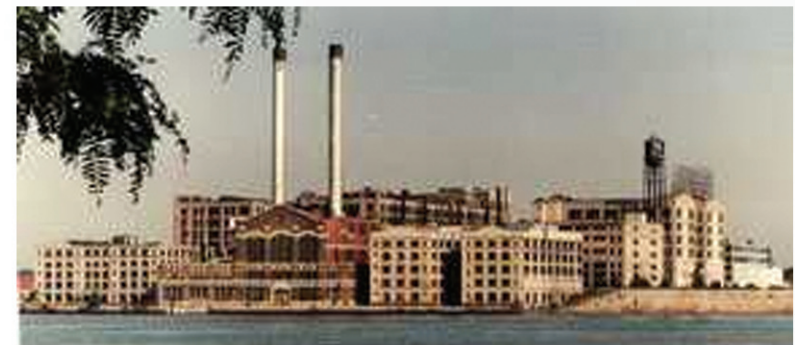
The UniRoyal Plant a year before its demolition
