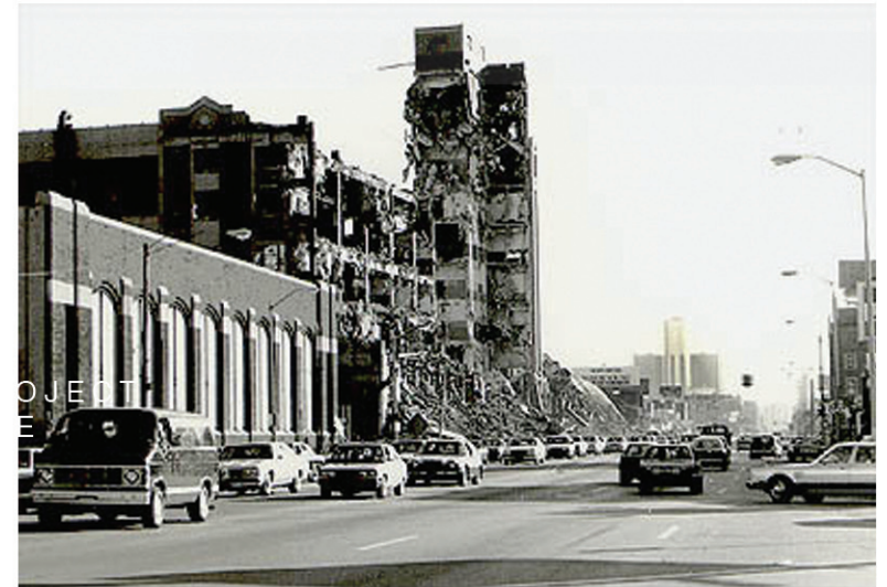
The UniRoyal Plant along Jefferson Ave. under demolition
