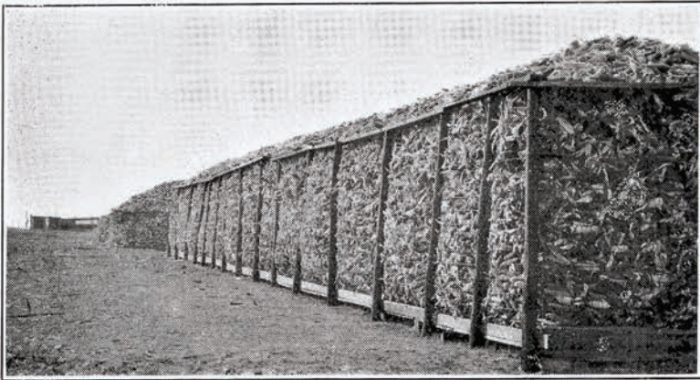
FIG. 23.—Much corn is stored in temporary wire or slat cribs. If the corn is placed on a wooden floor and shelled out during late winter or early spring, such cribs are practical and economical.
