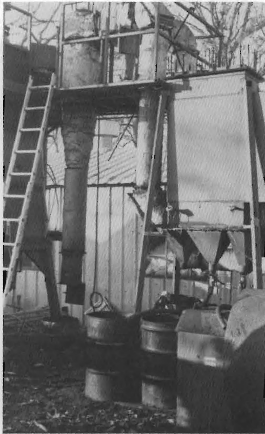
Figure 5. Close-up view of cyclone and condenser system--EES pyrolysis pilot plant.
