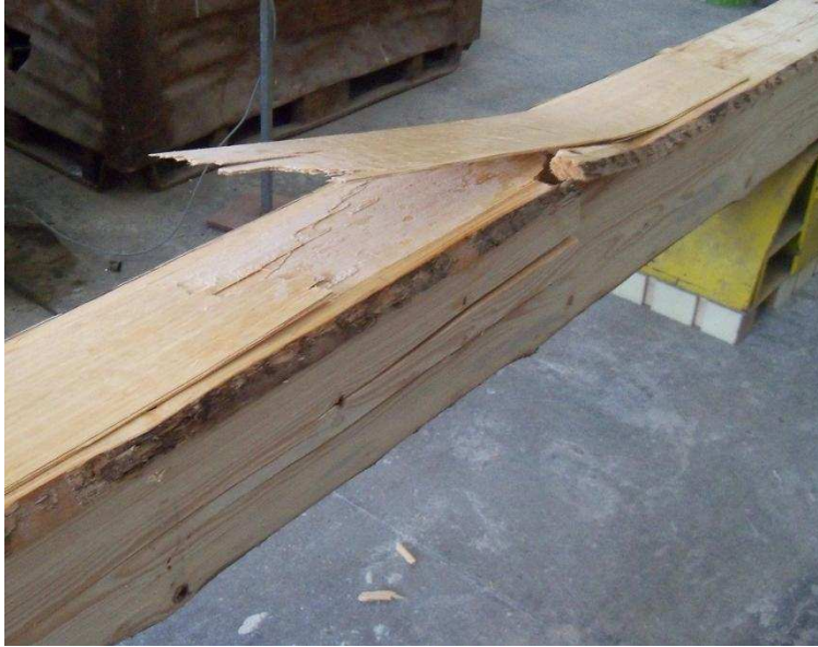
Figure 5. Flexural cracks and shear failure of reinforcement (bamboo reinforcement).
