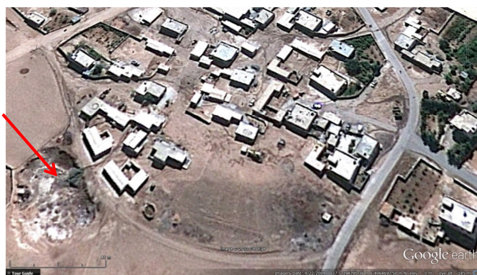
FIGURE 3-54: DUMPING PIT AT THE BASE OF KOULLIYE (LCP 50) 54
