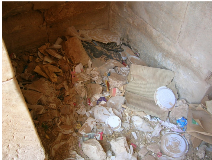
FIGURE 3-44: RUBBISH AT HALIBIYAH
