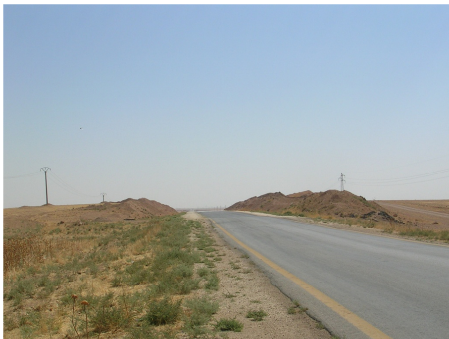
FIGURE 3-23: ROAD CUTTING THROUGH MOUND, ON THE ROAD FROM BRAK TO BEYDAR 30
