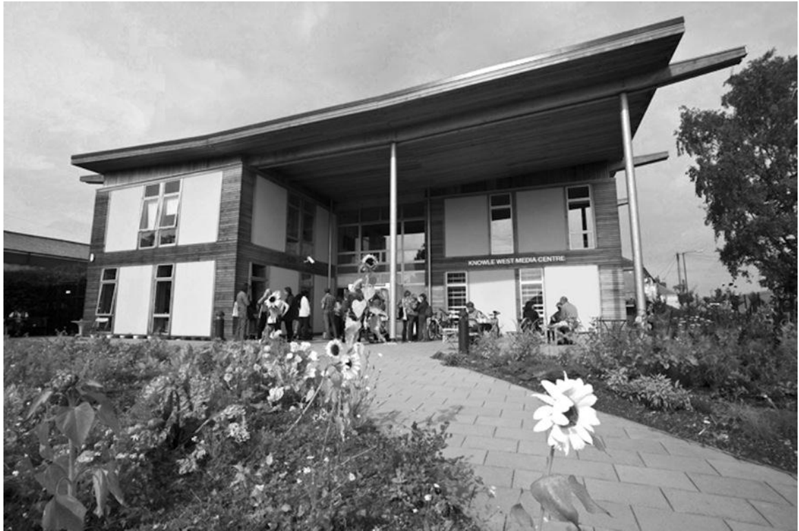
Figure 1. Knowle West Media Centre, Bristol, UK. The straw bale building has a computer lab, auditorium/gallery, sound studio, and office space for rent, among other amenities. Photo courtesy of Knowle West Media Centre.
