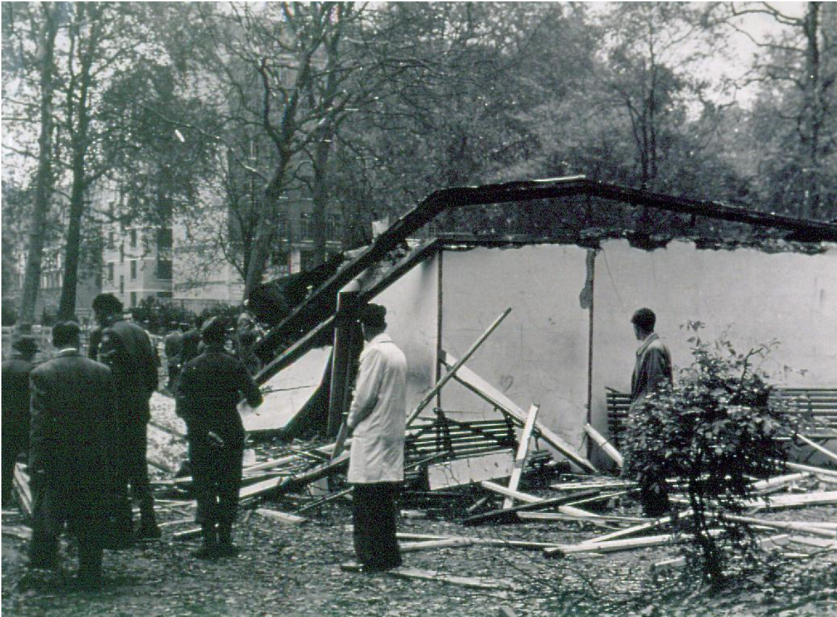
Figure 22. The central Pavilion destroyed by a bomb, 1944
