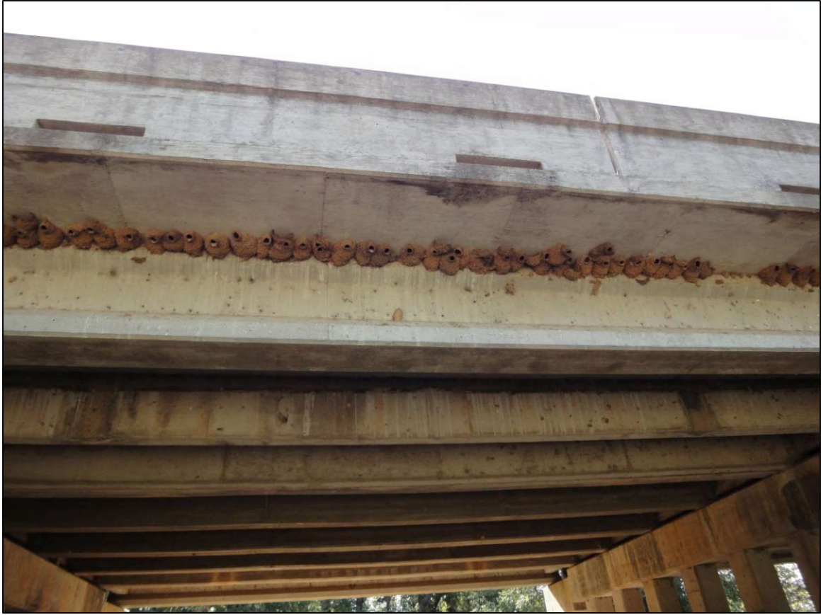
Cliff Swallow nests under bridge.
