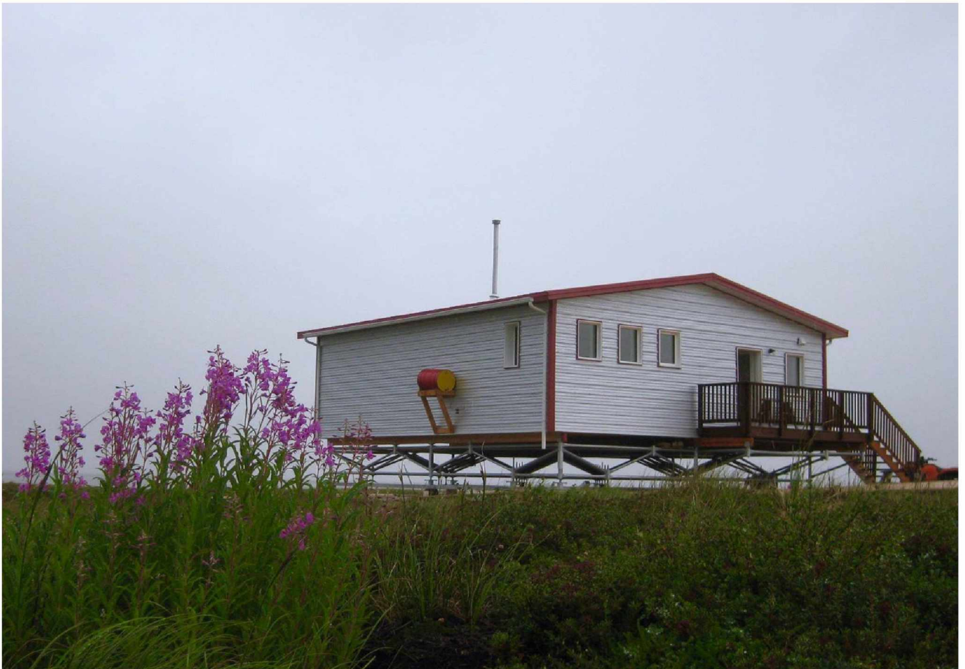
Completed CCHRC demonstration home in Mertarvik, Newtok's new community site
