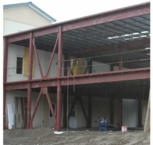
SNC addition under construction
