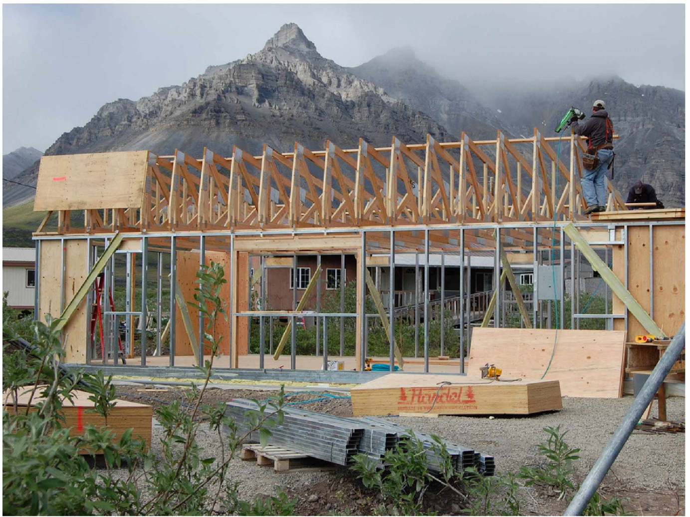
The first SNC prototype home under construction in Anaktuvuk Pass
