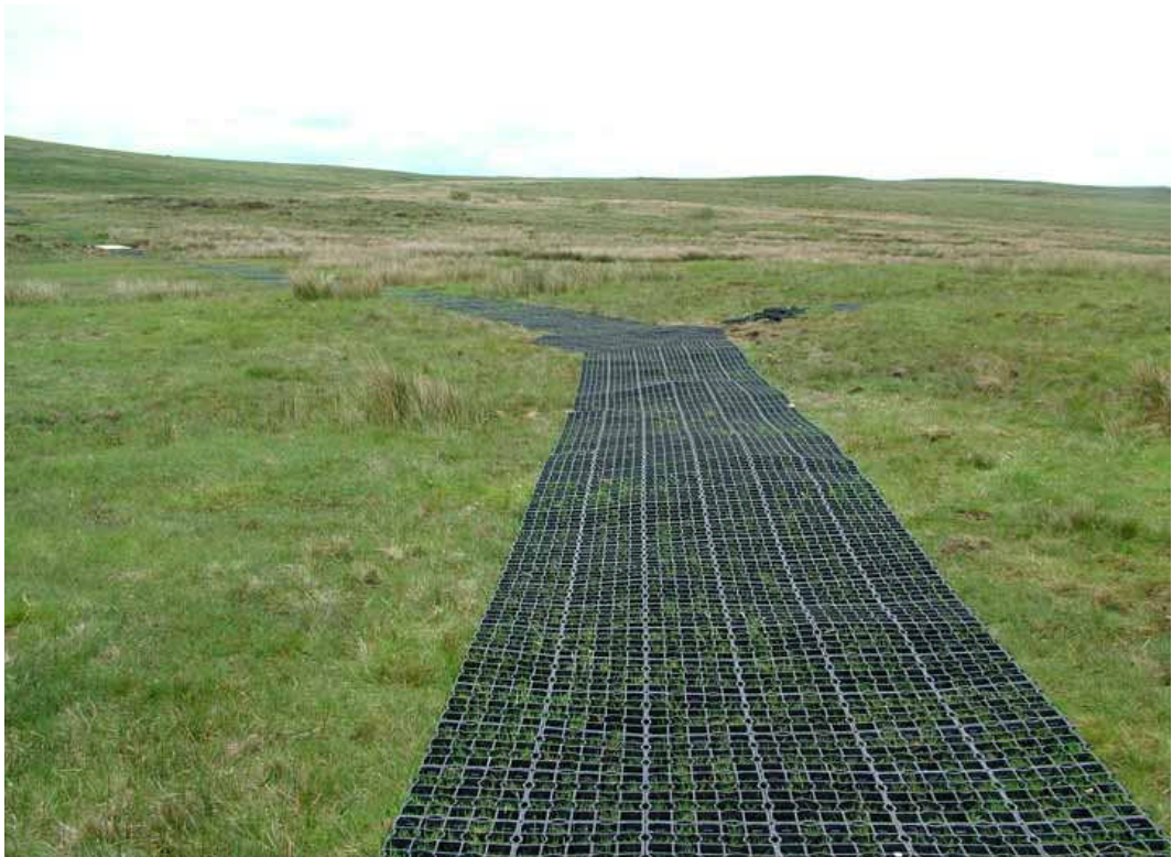
Figure 5.4. Eco-grid trail leading to Black Mountain. Photo courtesy of Belfast Hills Partnership.
