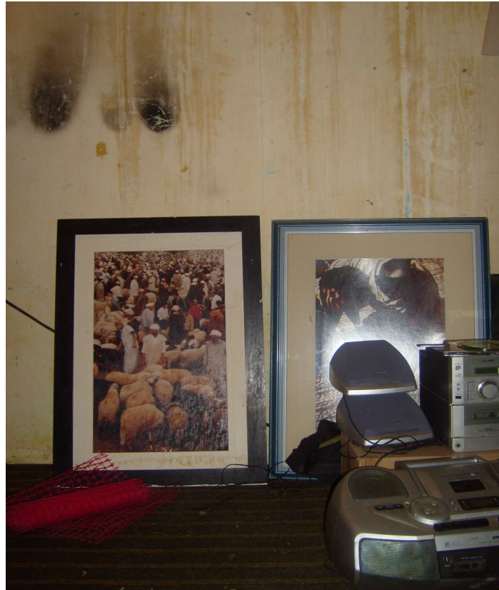
10. The Room above the Garage
