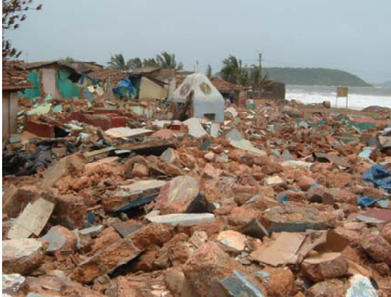
Figure 2-4: Baina after the demolition
