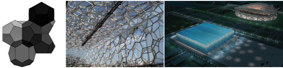
Figure 1: (a) The Weaire-Phelan structure (Drenckhan & Weaire, 2004) and (b) (c) Water Cube Beijing (Ingenia, 2007).
