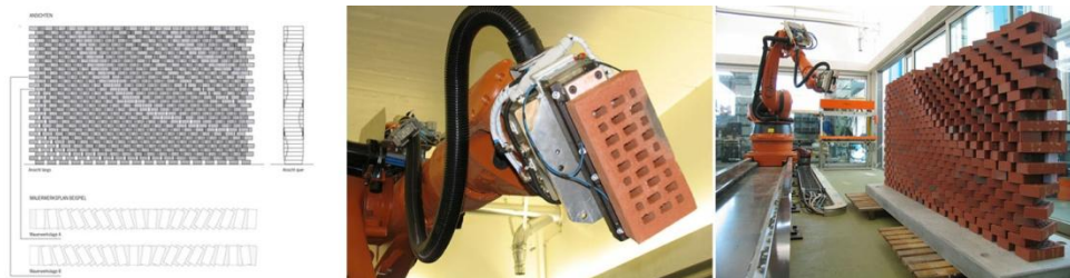
Figure 4: The programmed wall project by DFab Laboratory (Gramazio & Kohler, 2006).
