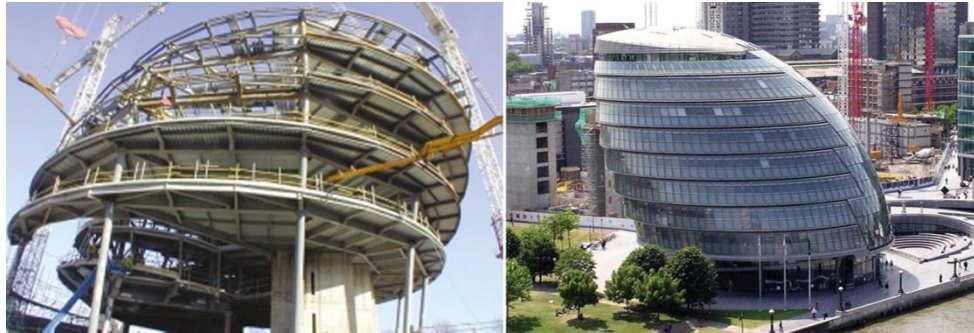
Figure 2: Greater London Authority by Foster and Partners (a) ( Constructing Excellence , 2003) (b) ( Oberholzer , 2006).
