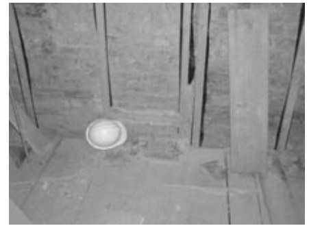
Fig. 2. At the LEVH, the demand for energy is reduced partly through a reduction in air infiltration. In this case, air infiltration is decreased through the installation of phenolic insulation panels, fixed on battens and sealed together with sealant foam.
