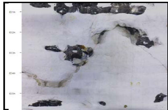
(d) Inclined fracture possibly solutionally enlarged at 47.2 m AOD
