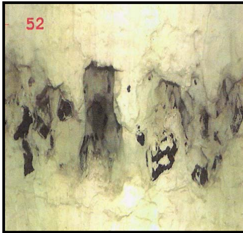
(a) Conduit, ~ 10 cm high at 52.2 m below datum/109.75 m AOD
