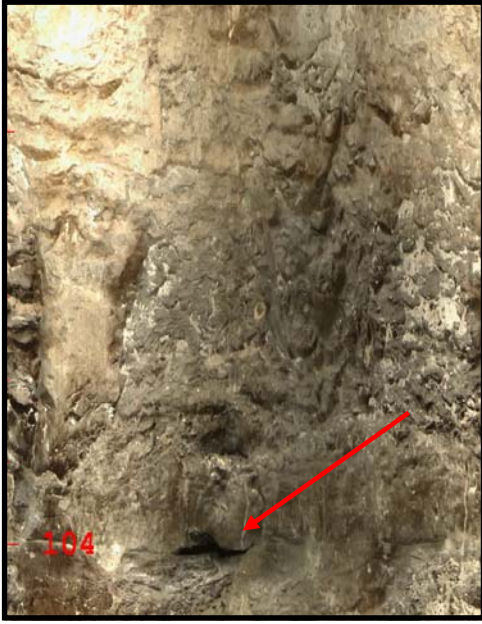
(a) Fracture at 45 m AOD (104 m below datum)
