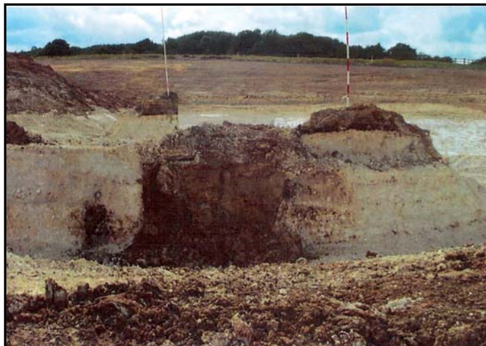
Figure 3.29: "Typical solution feature" at Chieveley, (Mott Macdonald, 2005)
