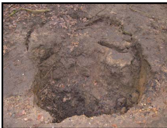
Figure 4.3: A newly formed sink point (hole diameter is approximately 1 m)
