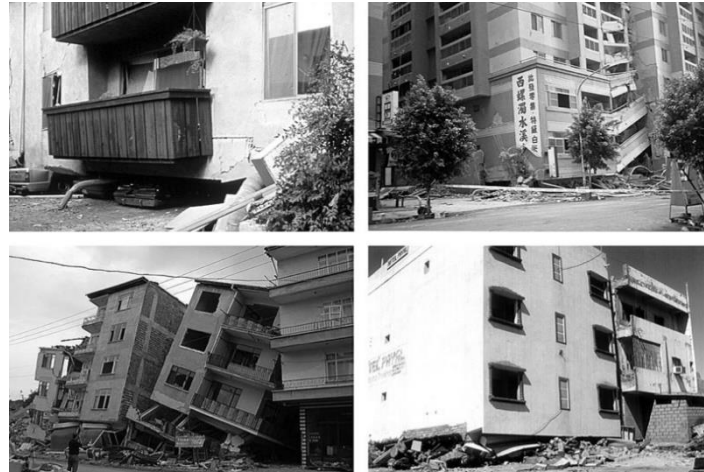
Figure 2. The soft storey failure mechanism
