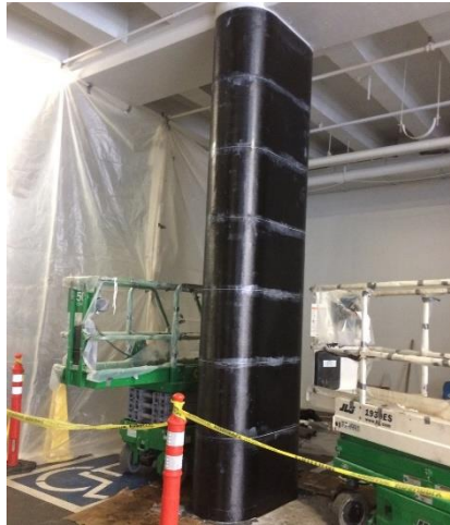
Figure 9. FRP jacketing of a column
