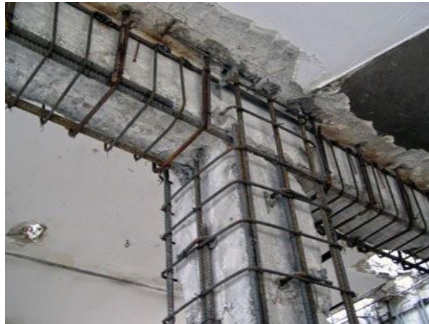
Figure 7. Reinforced concrete jacketing of a column and its supported beams
