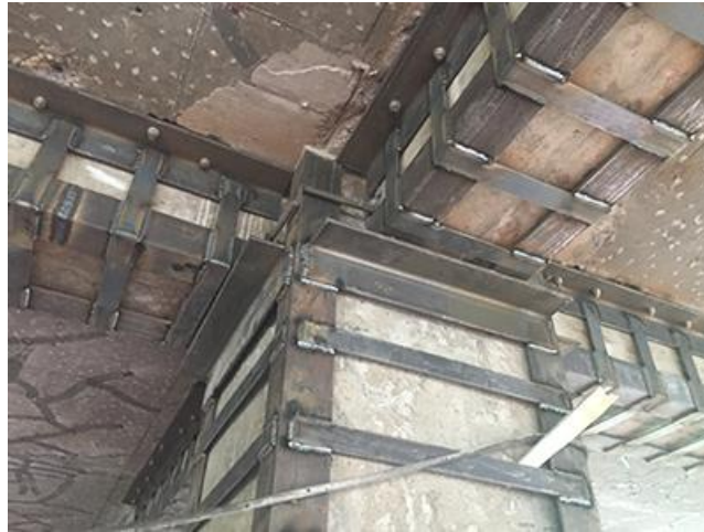
Figure 8. Retrofitting in RC members with steel plates
