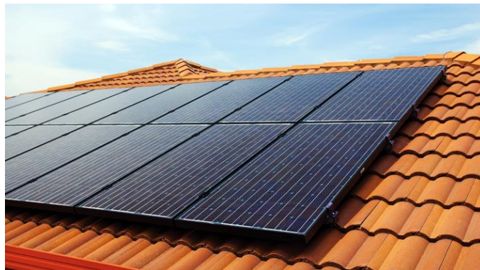
Figure 17. Solar panels installation on a residence's roof
