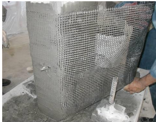
Figure 10. TRM jacketing of a column to be experimentally tested
